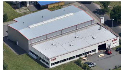
Plant II and Plant III
